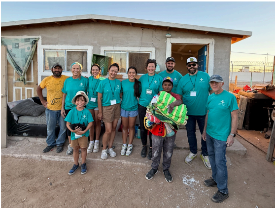
Celebrating after finishing the drywall and taping on a family's home.
