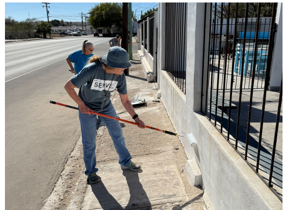
New paint for the walls of the Distribution Center.
